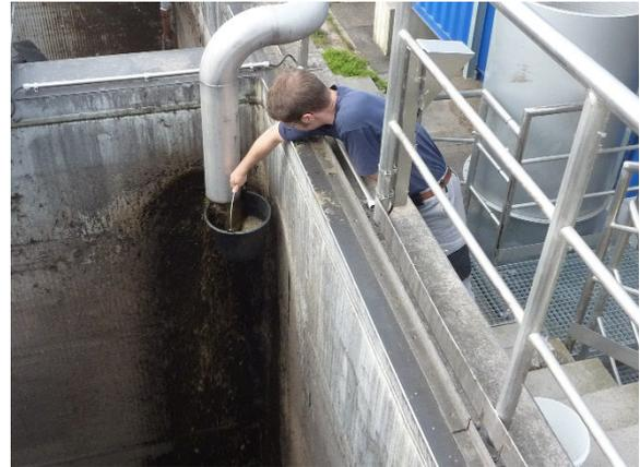
Fig. 18: Sampling of press fluid
